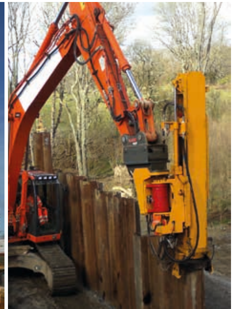
DX-SP DRIVING SHEET PILES
